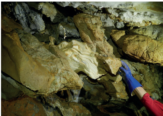
Figure 3: Corroded speleothem (ca. 650 ka old), filling gaps between block on the roof of Valdemino Cave (Photo Bartolomeo Vigna).
