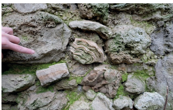
Figure 3: Speleothem fragments used for building the walls of a house at Ca' Monti (Photo by Veronica Chiarini).
